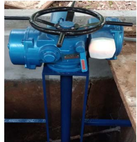
Figure 1.3. Block diagram of Actuator node. Figure 1.4. Electrical Actuator
